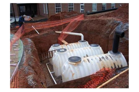
Cisterns collect rainfall from buildings and other impervious surfaces for reuse in campus buildings and landscapes. Underground drain pipes connect cisterns to their water source. A pump is then used to extract the water for use.
