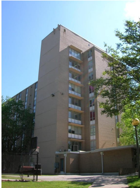
Figure 119. Oglethorpe House. (Source: University of Georgia)
