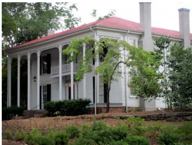
Figure 92. Treanor House. (Source: University of Georgia)
