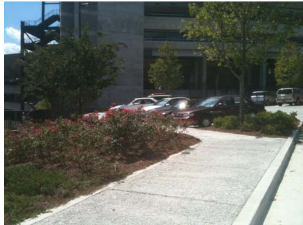
Porous Paving Sidewalk – Reed Plaza
