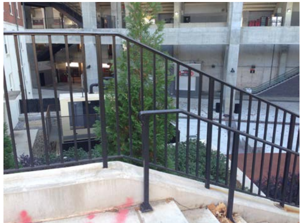
Handrails & Adjacent Guardrail – Reed Plaza
