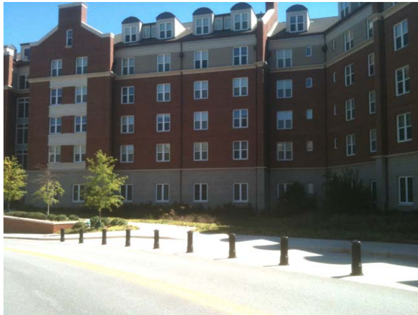
Security Bollards – Building 1516
