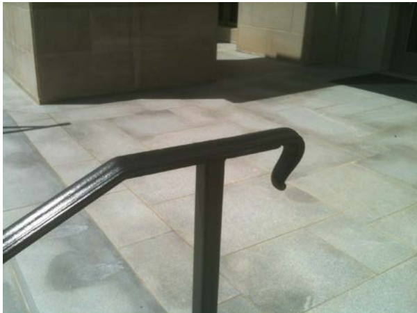
Handrails – Special Collections Library
