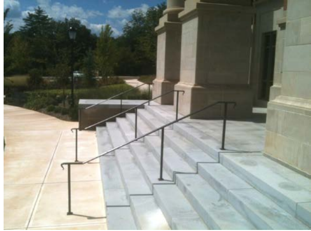
Stairs & Handrails – Special Collections Library
