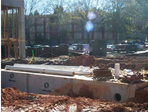
Underground Cistern – Paul D. Coverdell Center
