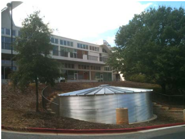
Above-Ground Cistern – Jackson Street Building
