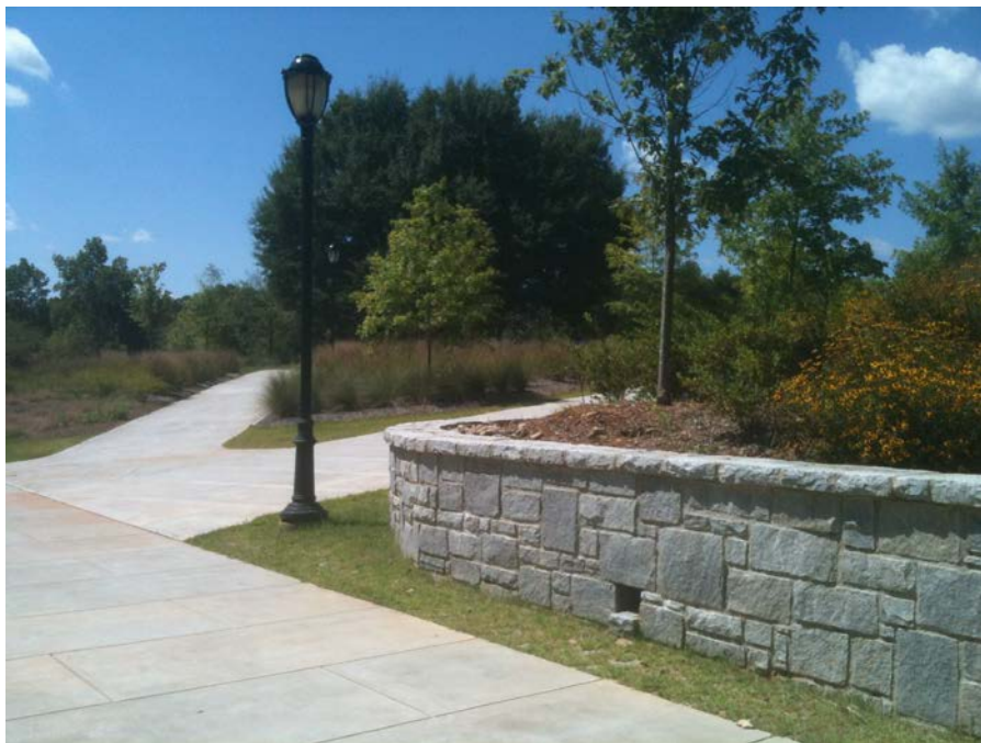
Granite Rubble Wall – Lamar Dodd School of Art & Georgia Museum of Art
