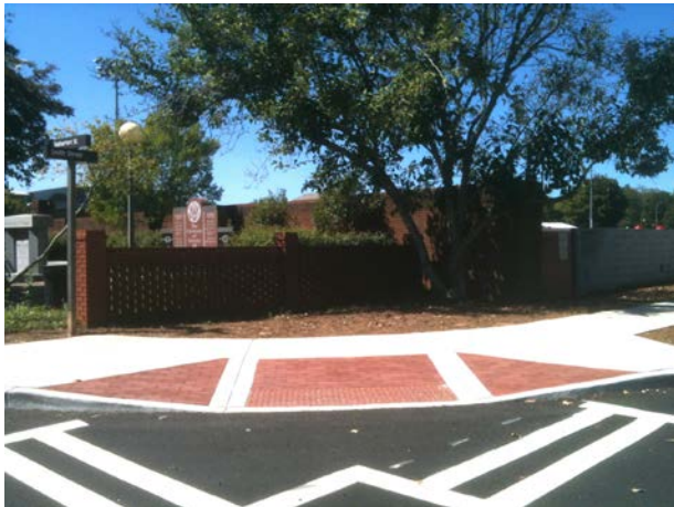
Crosswalks and Curb Cut with Truncated Domes – Stegeman Coliseum
