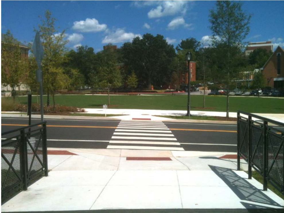
Crosswalk and Curb Cuts – Special Collections Library & Hull Street Deck
