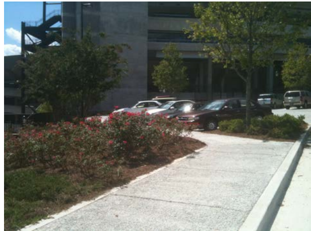
Porous Paving Sidewalk – Reed Plaza
