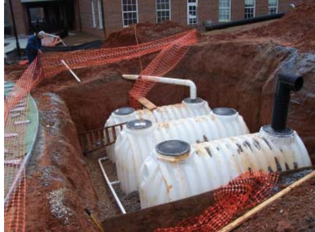
Underground Cistern – Miller Learning Center
