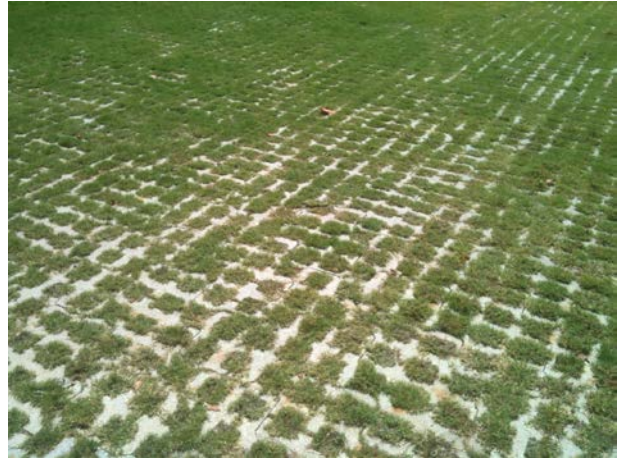
Grass Paving – Stegeman Coliseum
