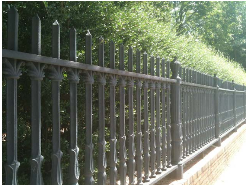
Cast Iron Fencing – Founders Garden
