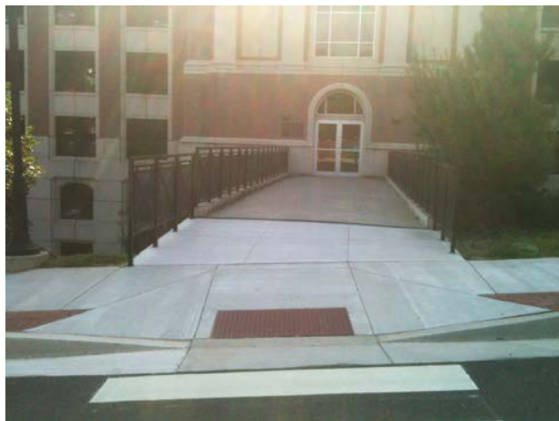
Curb Cut – Special Collections Library & Hull Street Deck
