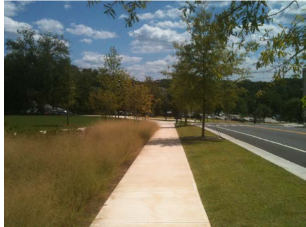
Sidewalk With Landscape Treatment – Special Collections Library
