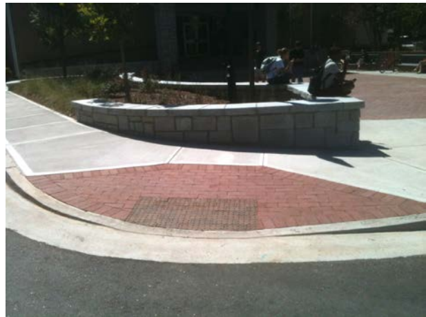
Curb Cut with Truncated Domes – Oglethorpe Dining Commons
