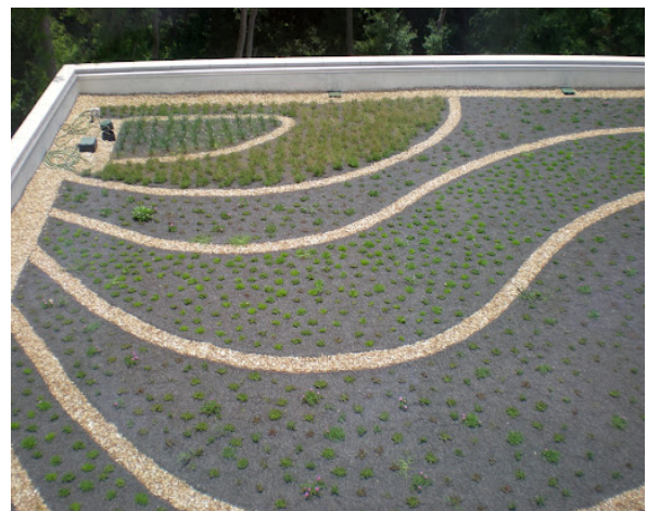
Green Roof – Lamar Dodd School of Art
