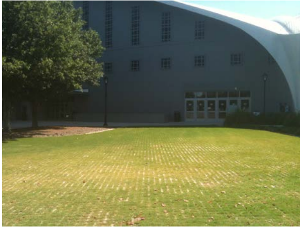
Grass Paving – Stegeman Coliseum
