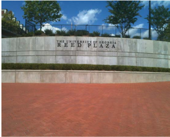
Brick Work – Reed Plaza
