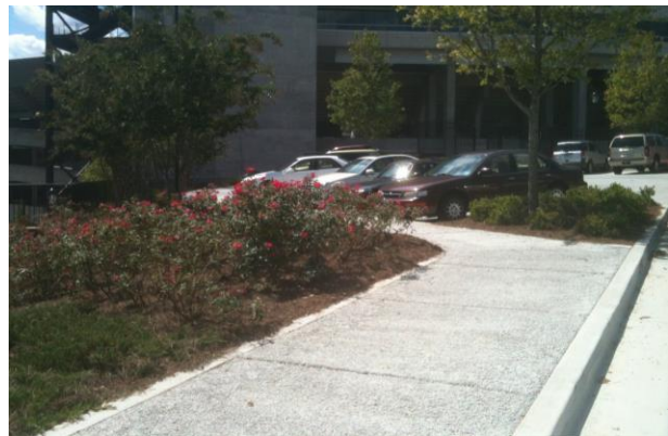
Porous Paving Sidewalk – Reed Plaza
