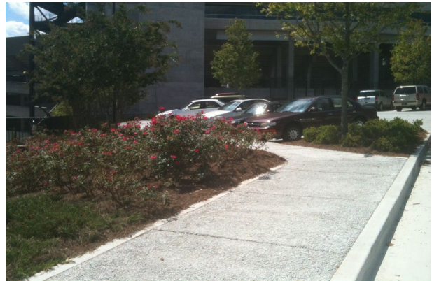
Porous Paving Sidewalk – Reed Plaza
