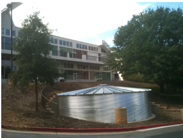
Above-Ground Cistern – Jackson Street Building
