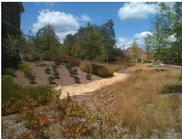
Bioswale – Special Collections Library
