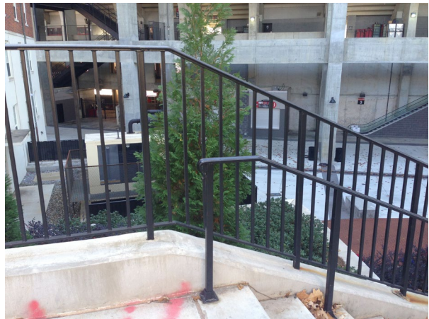
Handrails & Adjacent Guardrail – Reed Plaza
