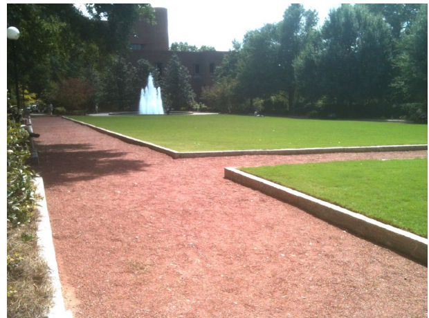
Granular Paving – Herty Field
