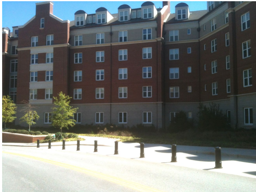
Security Bollards – Building 1516
