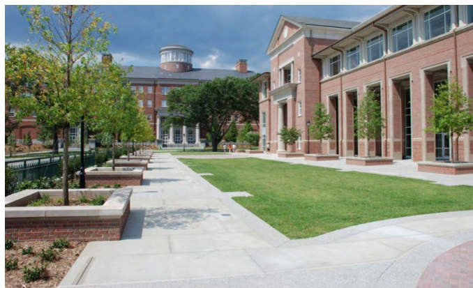
Green Roof – Tate Student Center
