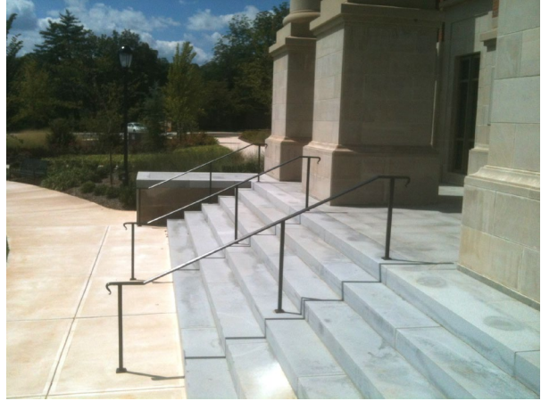
Stairs & Handrails – Special Collections Library
