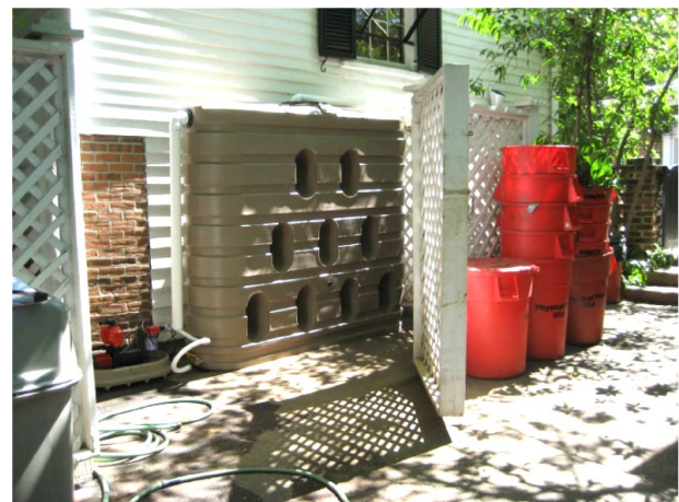
Above-Ground Cistern – Founders House
