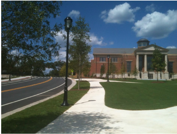
Sidewalk With Landscape Treatment – Special Collections Library
