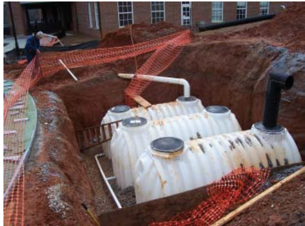
Underground Cistern – Miller Learning Center
