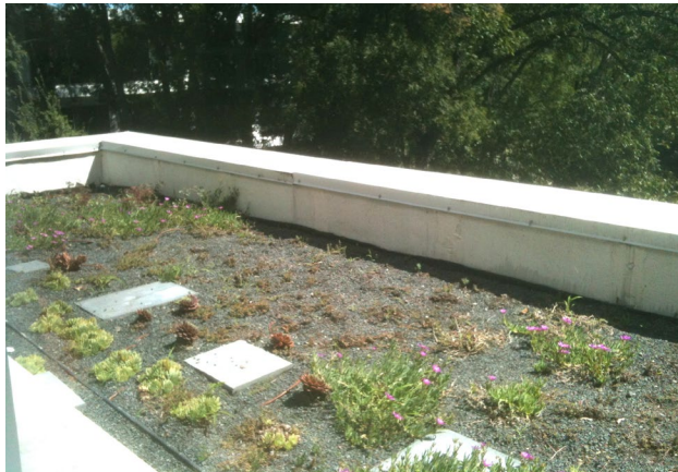
Green Roof – Robert C. Wilson Pharmacy Building
