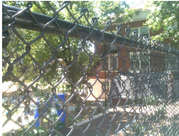
Chain-Link Fence – McPhaul Child & Family Development Center
