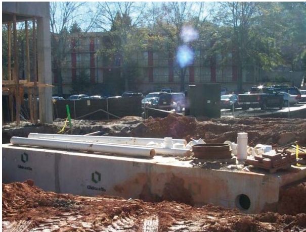
Underground Cistern – Paul D. Coverdell Center
