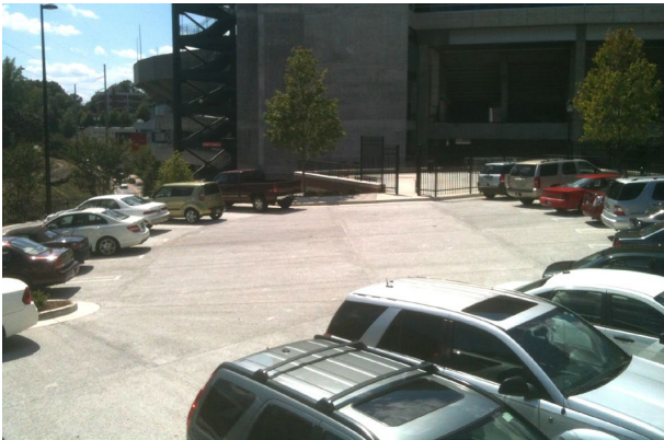
Porous Paving Parking Lot – Reed Plaza
