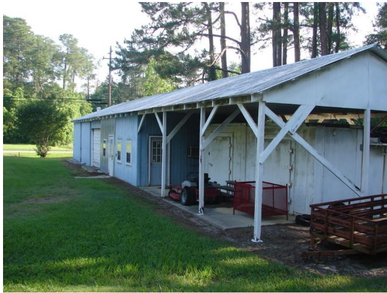
Figure 362. The Soils Shed is located at the western edge of the Tifton Campus south of Rainwater Road.
