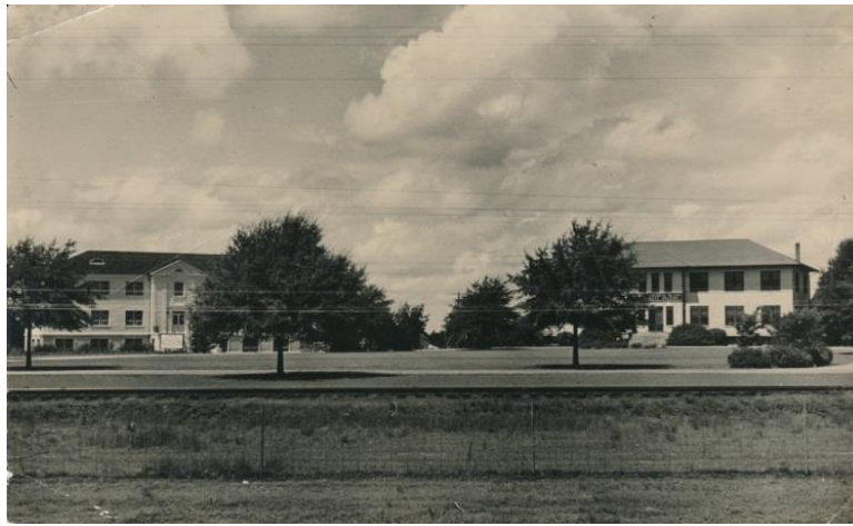
Figure 321. View of Animal and Dairy Science Building (left) and H. H. Tift Building (right), circa 1940s. (Source: University of Georgia Extension)
