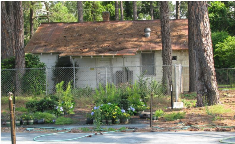
Figure 371. Laborers Cottage A.
