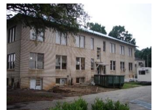
Figure 332. Rear facade, H. H. Tift Building.
