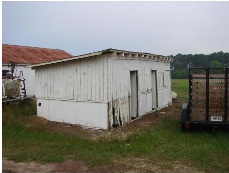
Figure 384. The Fuel House.
