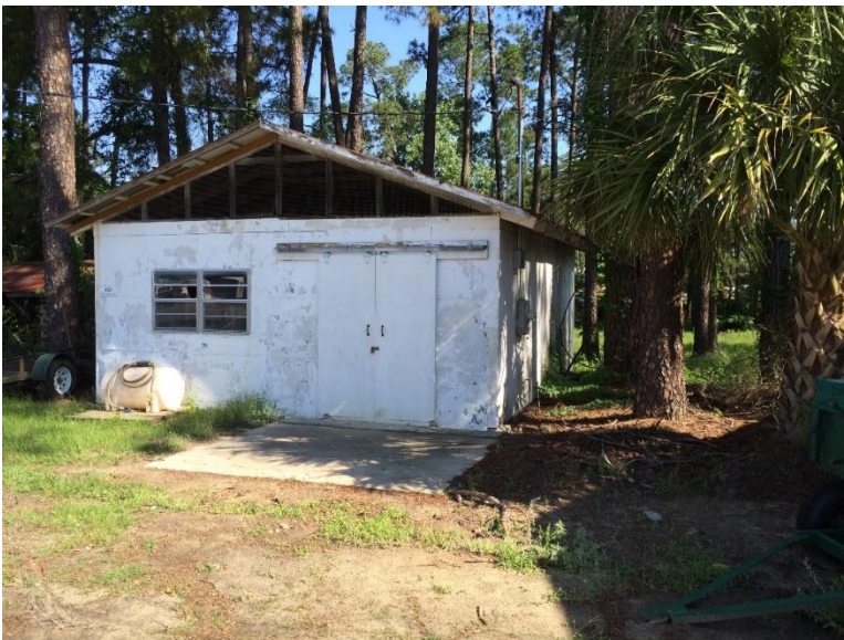
Figure 367. The Plant Pathology Growth Chamber.
