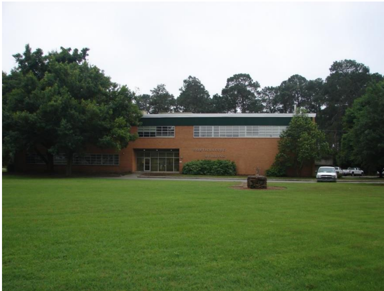
Figure 336. Front view of the Horticulture Building, 2015.
