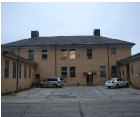
Figure 329. Rear view, Old Administration Building.
