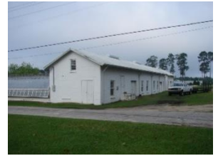
Figure 342. Side view of Greenhouse no. 2.
