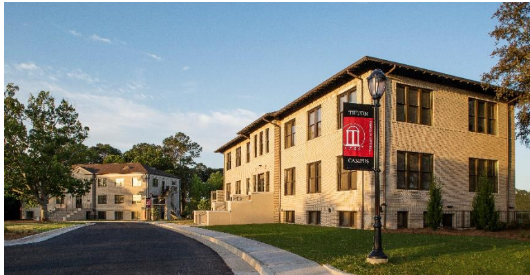
Figure 333. View of Animal and Dairy Science Building (left) and H. H. Tift Building (right). (Source: University of Georgia, Office of the University Architects)
