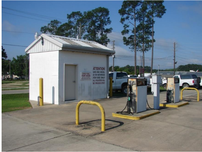
Figure 340. Fuel Monitoring Building.
