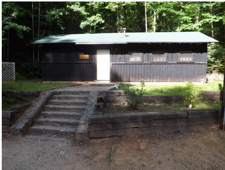
Figure 488. Camp Wahsega boys' bathhouse.
