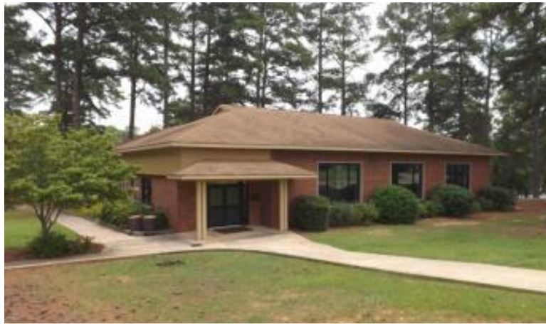
Figure 451. The Hastings Building.
