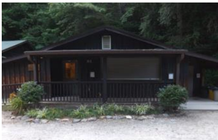
Figure 481. Camp Wahsega craft food storage building.
