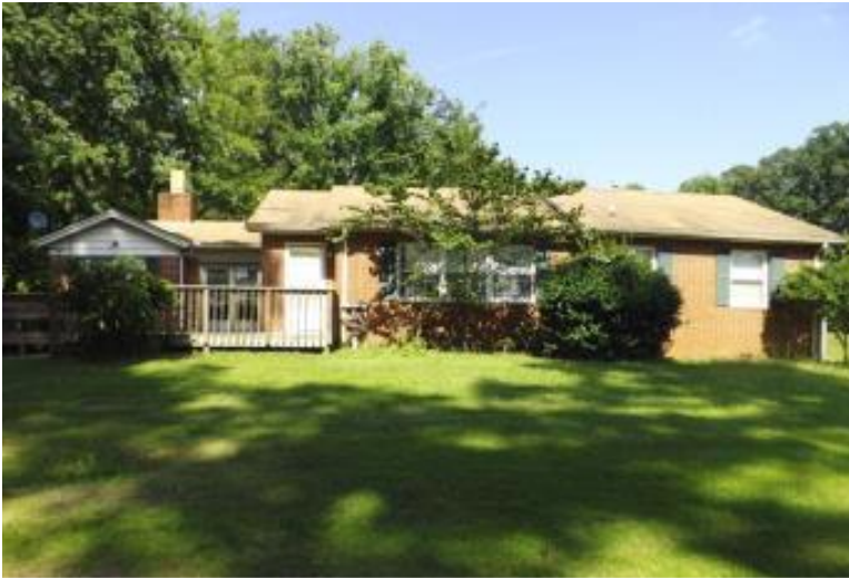
Figure 463. The Resident Jenkins building.
