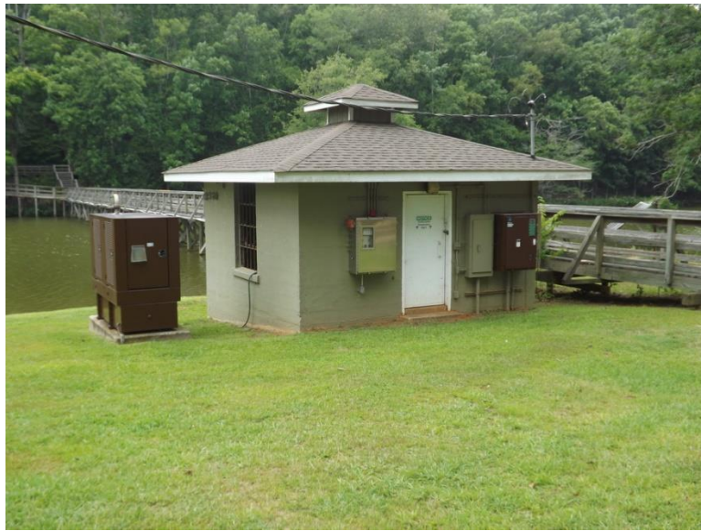
Figure 470. The Sewerage lift station.
