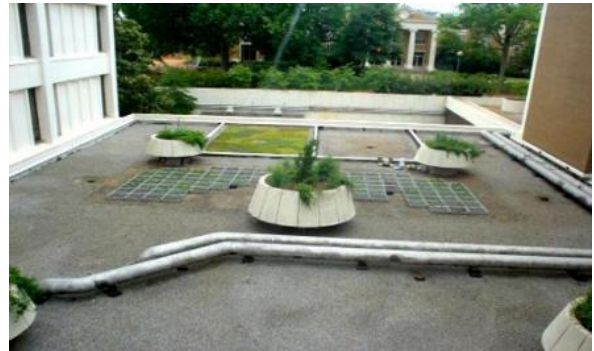
Green Roof – Science Library
