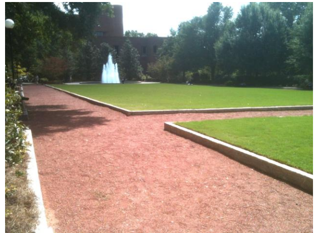
Granular Paving – Herty Field
