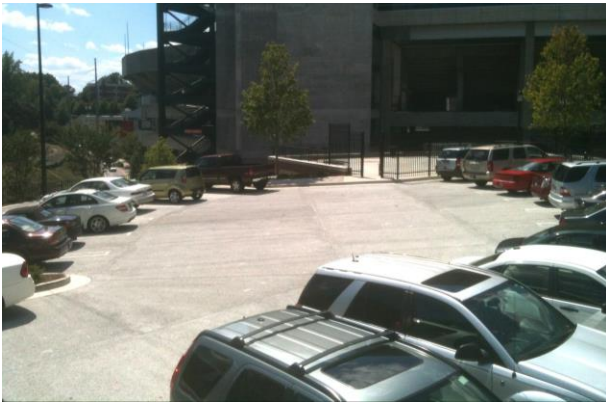
Porous Paving Parking Lot – Reed Plaza
