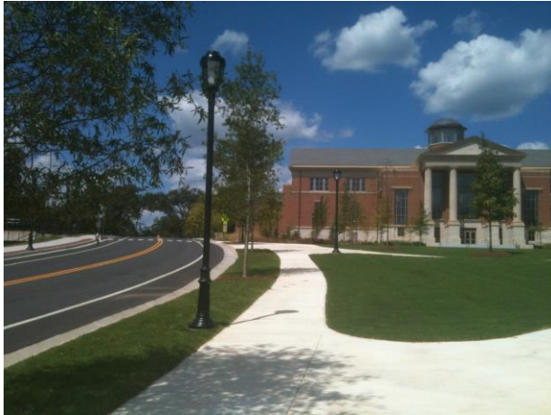
Sidewalk With Landscape Treatment – Special Collections Library
