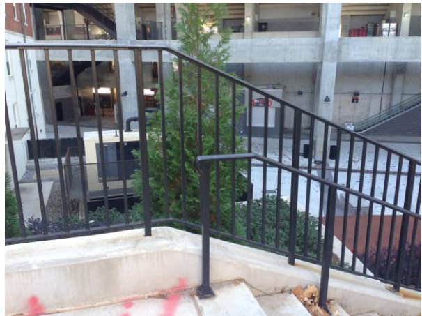
Handrails & Adjacent Guardrail – Reed Plaza
