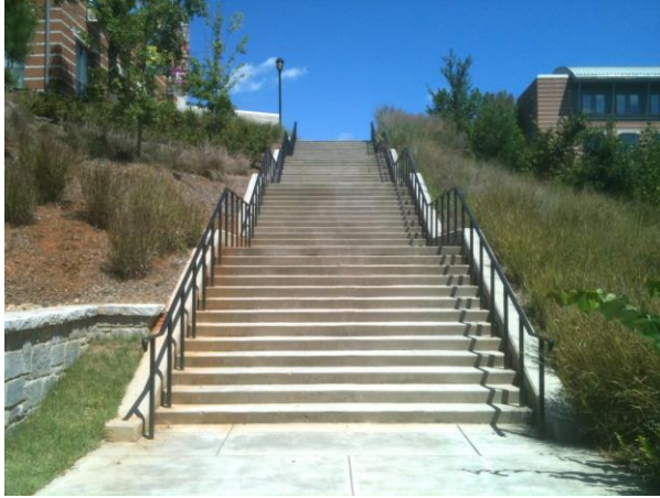
Stairs & Handrails – Lamar Dodd School of Art & Georgia Museum of Art
