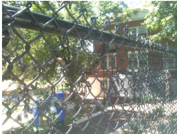
Chain-Link Fence – McPhaul Child & Family Development Center
