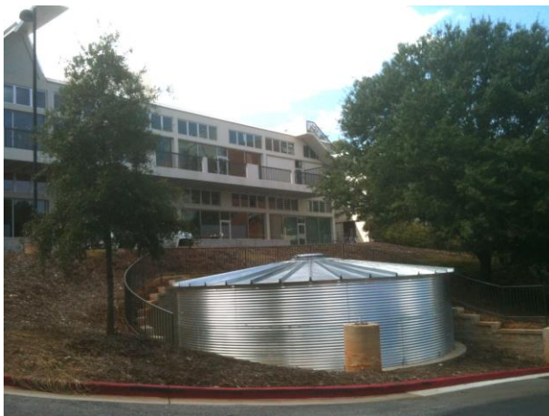
Above-Ground Cistern – Jackson Street Building
