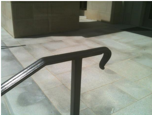
Handrails – Special Collections Library
