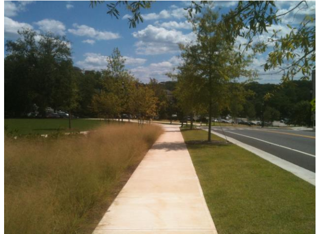
Sidewalk With Landscape Treatment – Special Collections Library
