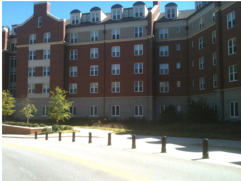
Security Bollards – Building 1516
