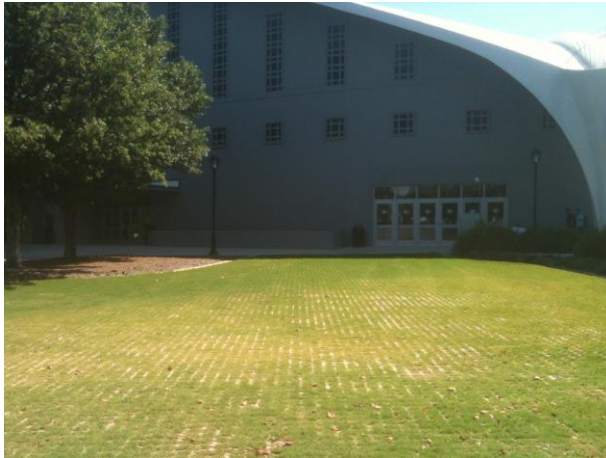
Grass Paving – Stegeman Coliseum
