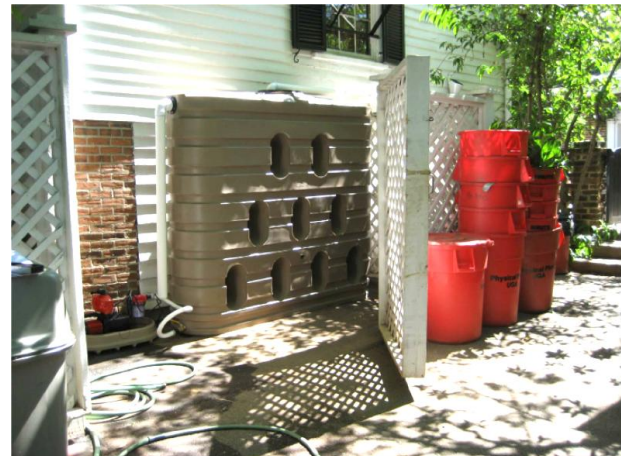
Above-Ground Cistern – Founders House
