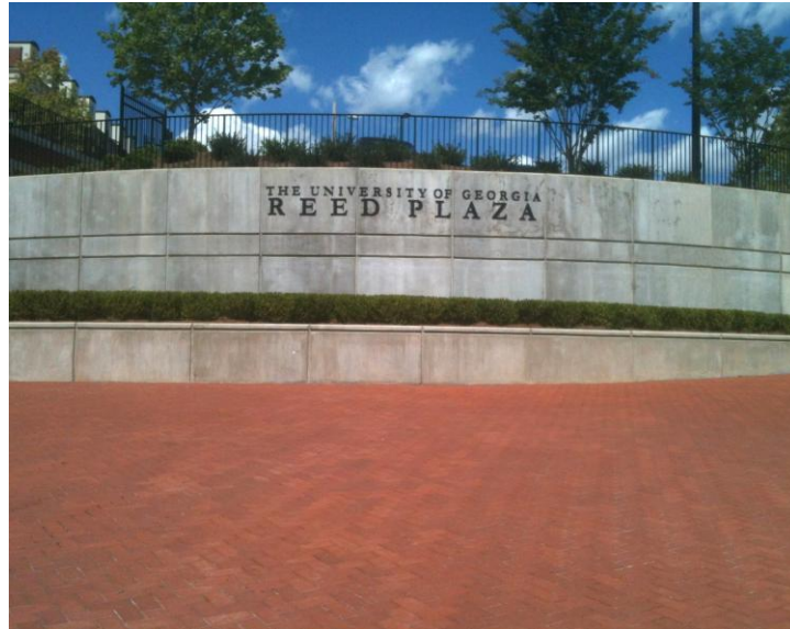
Brick Work – Reed Plaza
