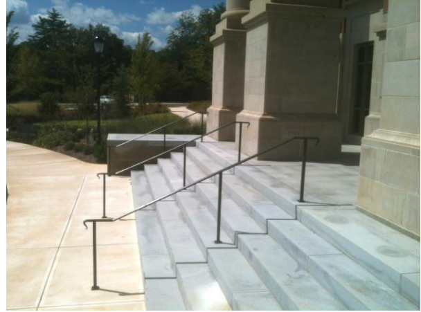
Stairs & Handrails – Special Collections Library
