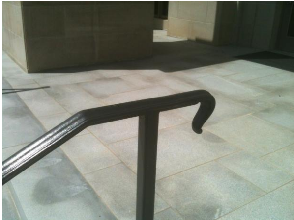
Handrails – Special Collections Library
