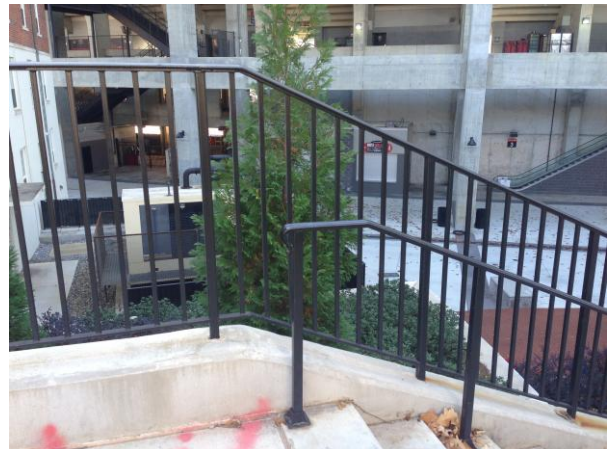
Handrails & Adjacent Guardrail – Reed Plaza
