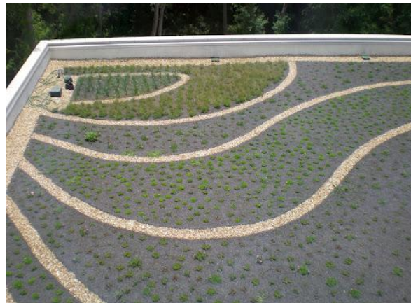
Green Roof – Lamar Dodd School of Art
