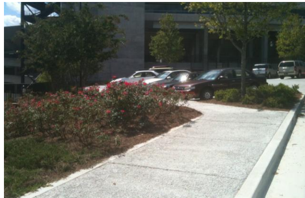
Porous Paving Sidewalk – Reed Plaza
