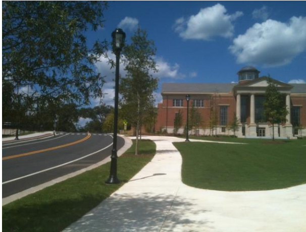
Sidewalk With Landscape Treatment – Special Collections Library
