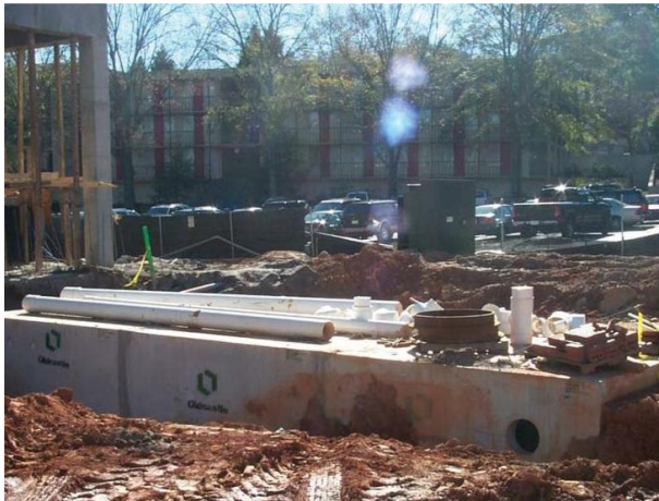
Underground Cistern – Paul D. Coverdell Center
