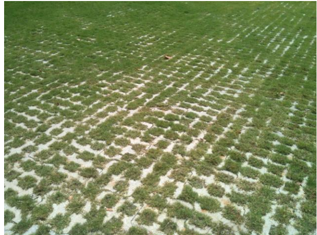
Grass Paving – Stegeman Coliseum
