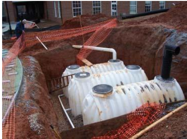
Underground Cistern – Miller Learning Center
