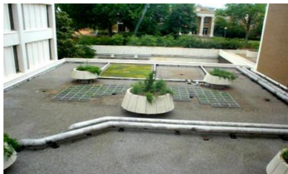
Green Roof – Science Library
