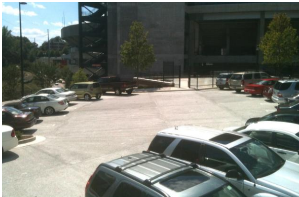
Porous Paving Parking Lot – Reed Plaza
