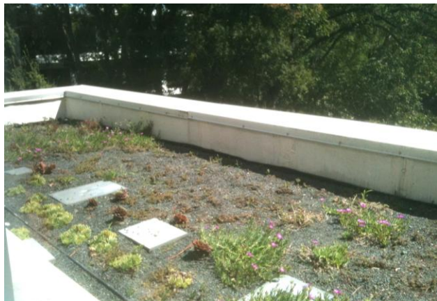
Green Roof – Robert C. Wilson Pharmacy Building
