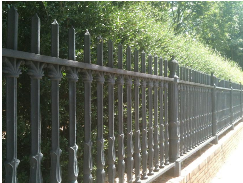
Cast Iron Fencing – Founders Garden
